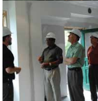
Waterloo North Hydro staff tour REEP House with Ben Barclay: Albert Singh, VP Finance and CFO, John Janzen, Customer Accounts Supervisor, and Rene Gatien, President.
